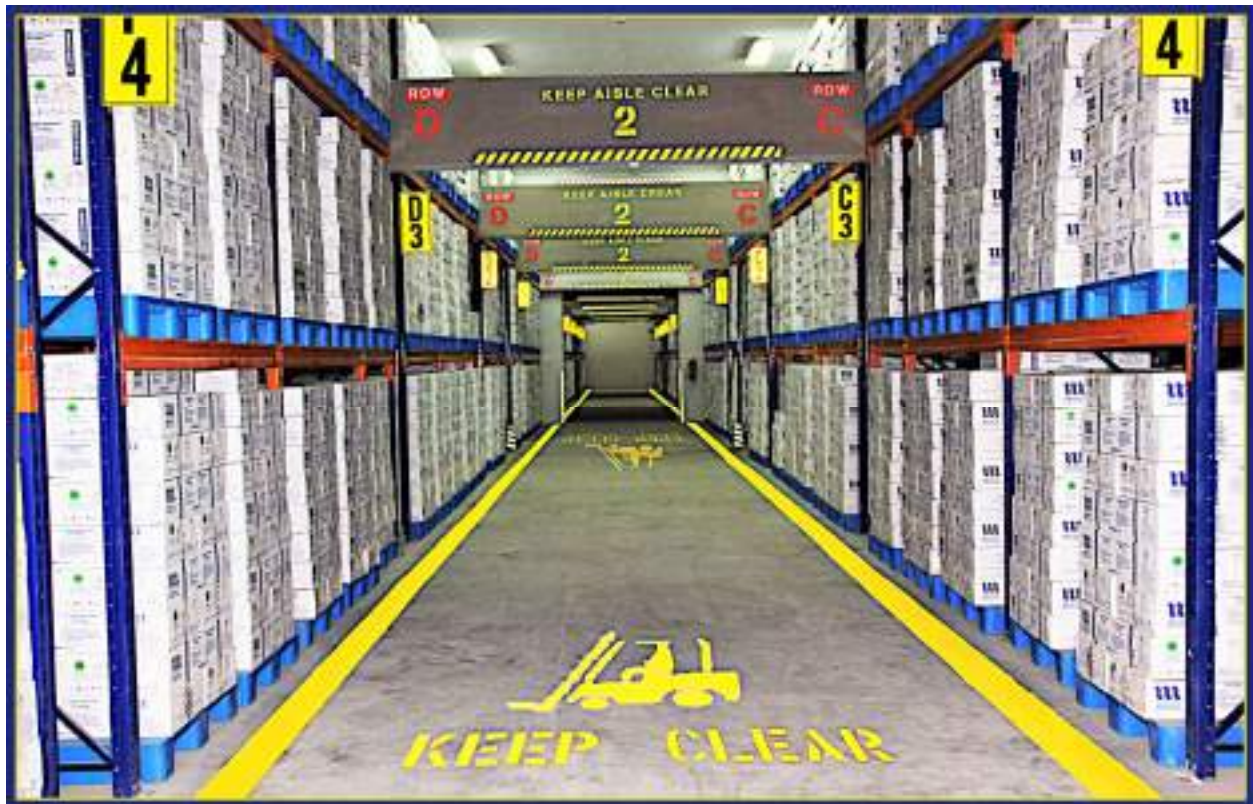
Figure 40. Pallet Racking System at Warehouse
