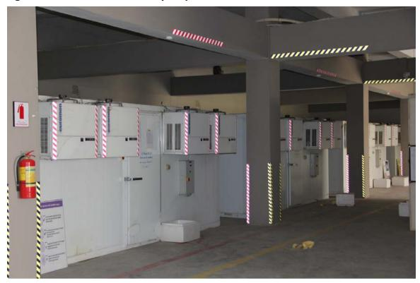
Figure 19. Cold Room 50 m3 Capacity at Federal EPI Store
