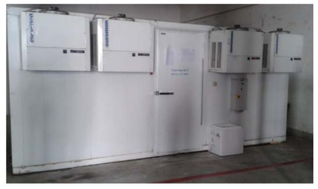
Figure 20. Freezer Room 50 m3 Capacity at Federal EPI Store
